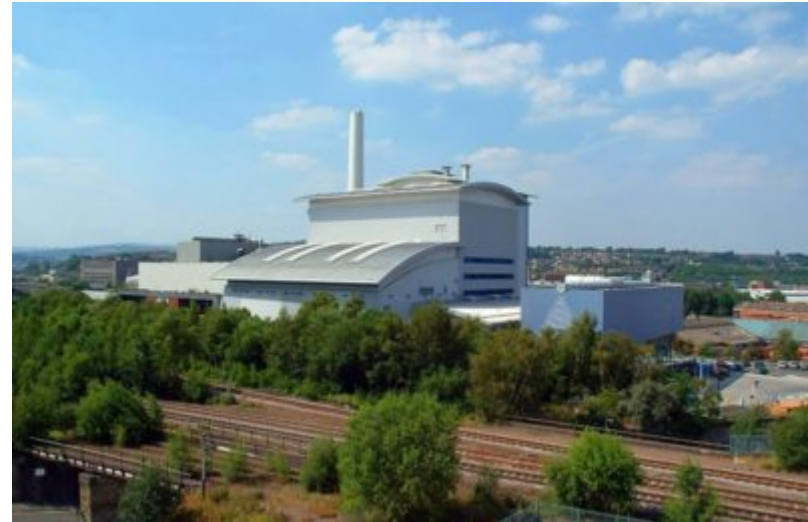
Veolia Energy Recovery Facility; Bernard Road, Sheffield.
